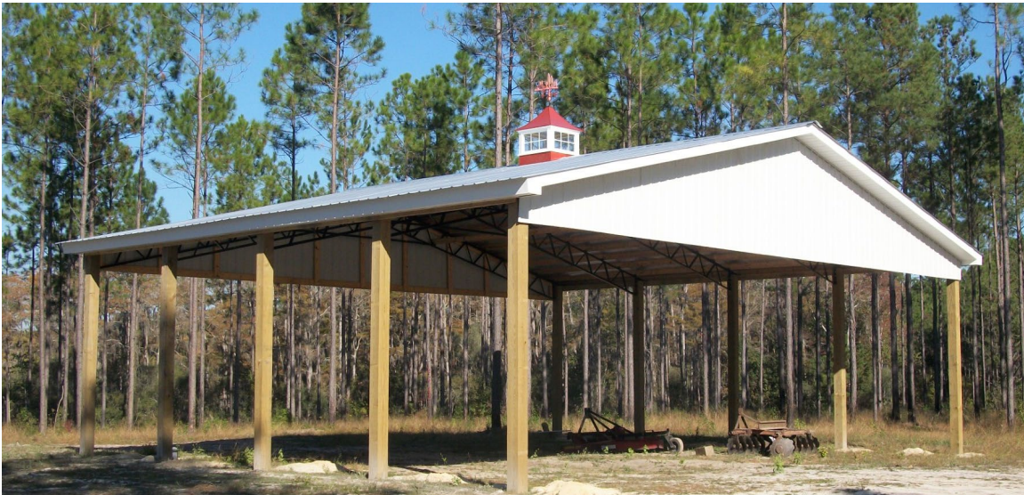
Pole barn example provided by sponsor
